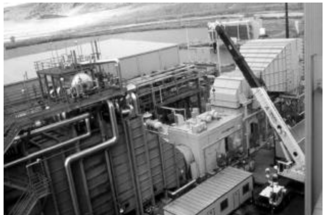
Figure 6. General Electric MS6001FA gas turbine (right) connected to HRSG (left).
