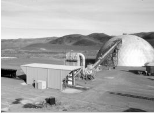
Figure 3. Coal unloading and coal storage dome. A 20-day supply of coal is kept in this 250-foot diameter
